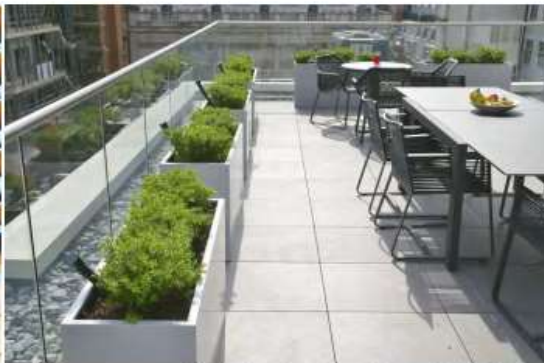
Roof terrace: Structural glass balustrade with stainless steel handrail Porcelain paving tiles
