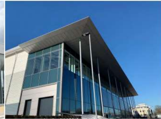
Overhang and curtain walling
