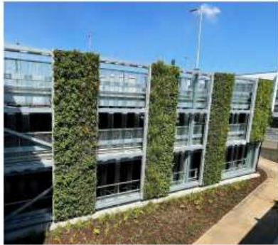
Car park hit-and-miss glass panels and green wall (to match Bedford Avenue carpark) Glass panels: Profilit glass
