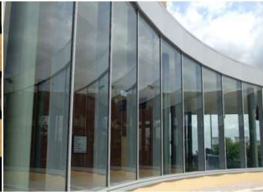
Faceted curtain walling to main entrance
